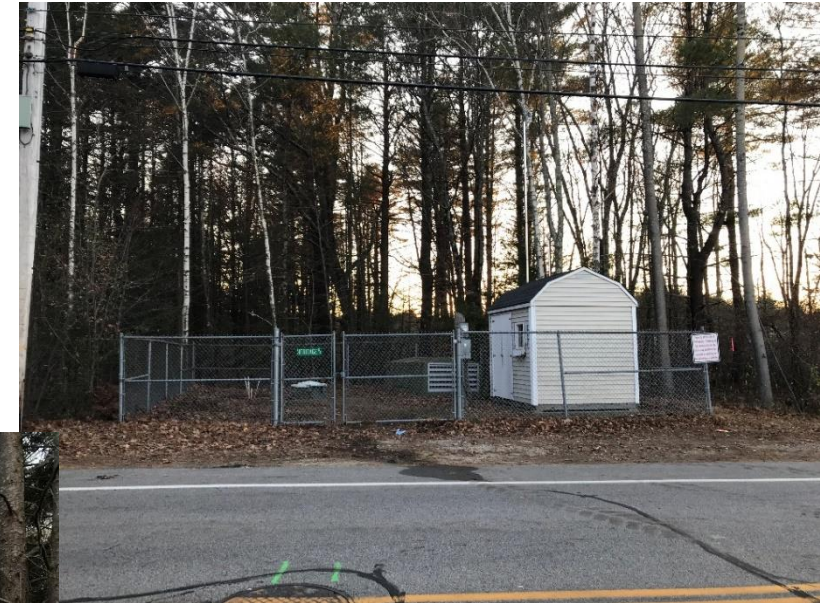
Photo: Heritage Ave Pump Station
